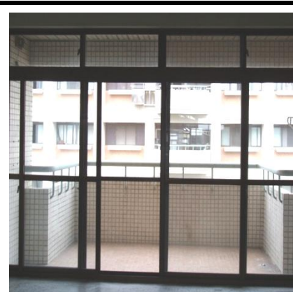
陽台 (○) Balcony clean & neat
